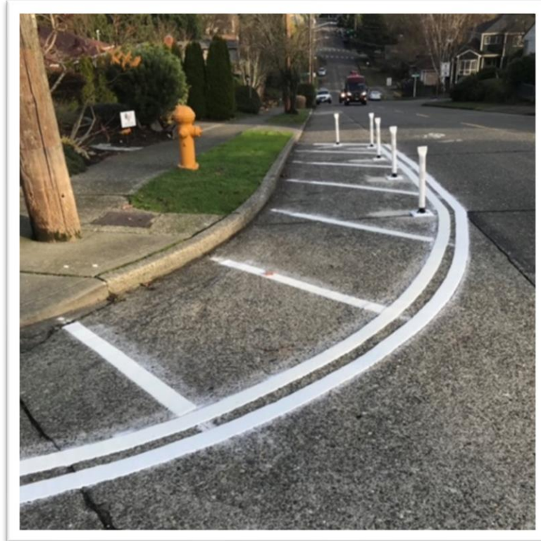
Crews installed 6 paint and post projects at three locations in the Fauntleroy neighborhood, and two at Marginal Way PI and 17 th Ave SW.
